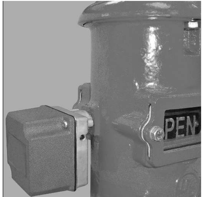
13. Use the operating wrench to check for proper operation of the indicator. Verify that the "OPEN" target plate is completely visible in the window when the valve is in the fully open position. Verify that the "CLOSED" target plate is completely visible in the window when the valve is in the fully closed position.
