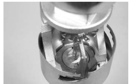
CORRECT ENGAGEMENT FOR MODEL V36 CONCEALED/RECESSED WRENCH
